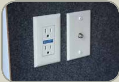
110v outlet and cable outlet conveniently located in the pass-thru storage area.
