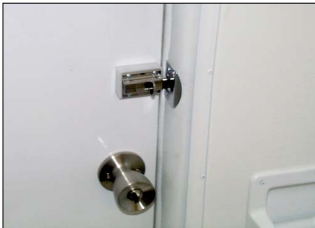
Slide Bolt that Operates Vacant / Occupied Indicators
