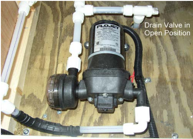
Fresh Water Pump (exposed)
