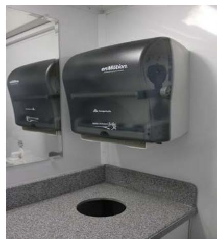
Paper Towel Dispenser and Trash Disposal Access
