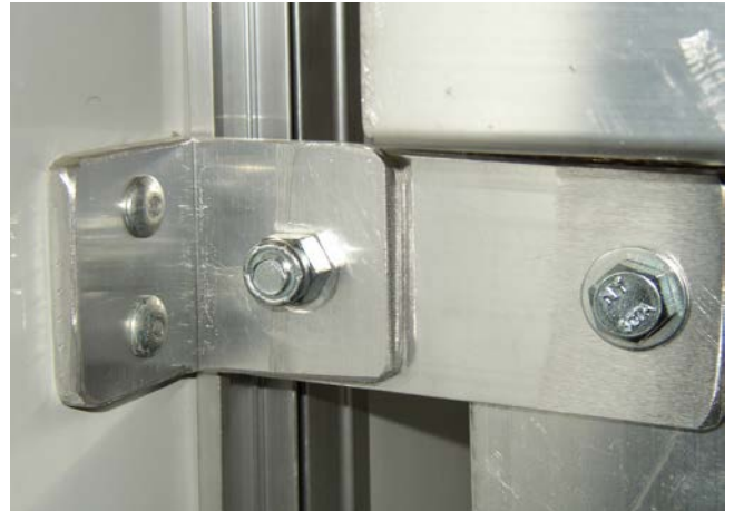
Bracket - Holds Porch in Retracted Position
