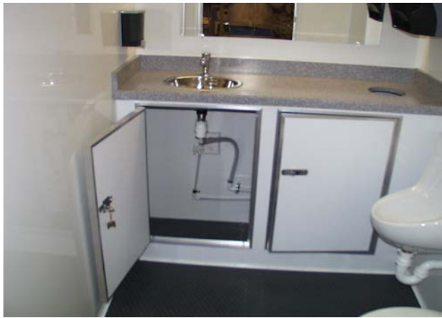
View of Sink Drain Set-Up Inside Lockable Base Cabinet
