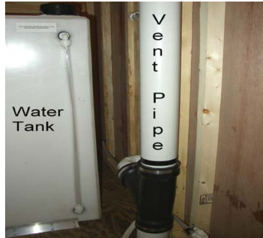
View of Vent Pipe and Fresh Water Tank with Level Indicator Tube
