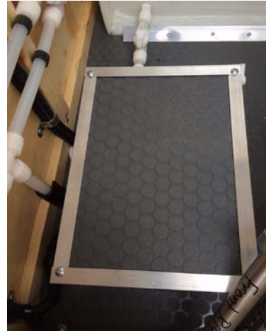
Fresh Water Pump with Cover
