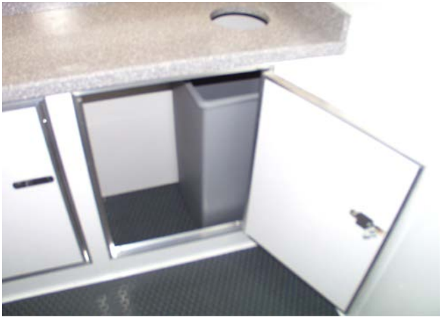
View of Trash Collection Receptacle In Locking Base Cabinet
