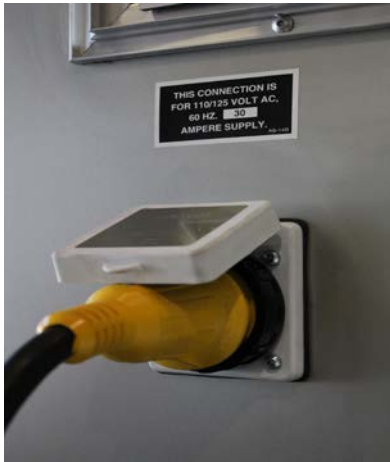
Exterior RV Style Electrical Cord Hook-Up
