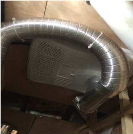
Roof A/C and Ducts
