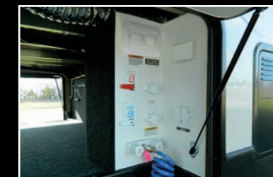
Convenience center with winterization, water heater by-pass and black tank flush
