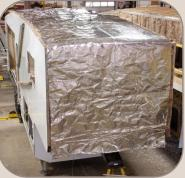
Triple layered residential insulation is installed including a Radiant Thermo-Foil, with an R-value of 38, which is wrapped underneath the front cap.
