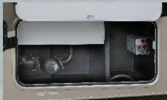
HEATED AND ENCLOSED Heated/enclosed utility station uses warm air from the furnace to protect tanks and valves. (N/A 2251 SLE)
