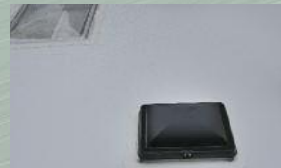
FIBERGLASS ROOF Durable, easy to clean (R-18) crowned fiberglass sheds water and doesn't cause black streaks like a rubber roof.
