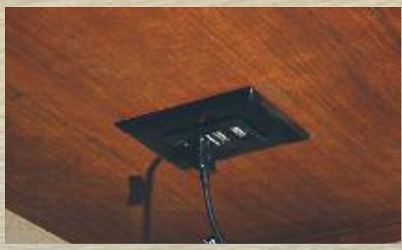
USB CHARGING STATION 12V 4-port USB charging station (Living room/bedroom)
