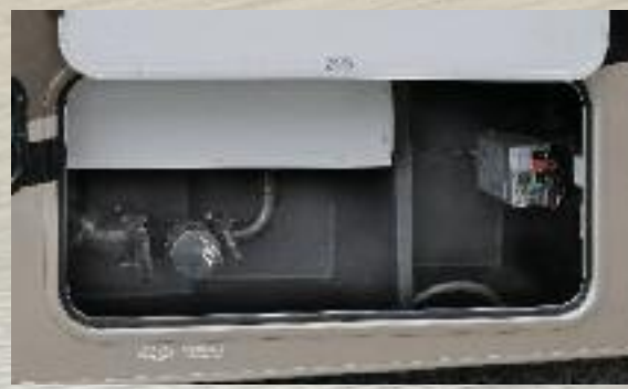
HEATED AND ENCLOSED Heated/enclosed utility station uses warm air from the furnace to protect tanks and valves. (N/A 2250 SLE)
