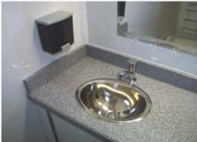
Sink and Soap Dispenser
