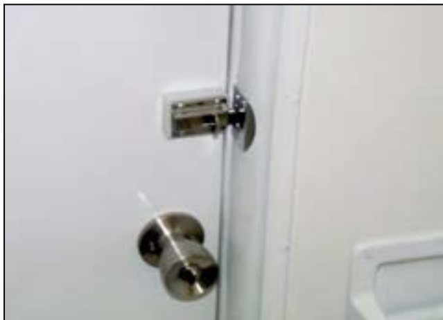
Slide Bolt that Operates Vacant / Occupied Indicators
