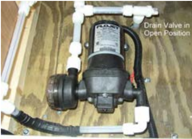
Fresh Water Pump (exposed)
