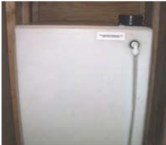
On-Board Fresh Water Tank Showing Fill Cap on Top of Tank
