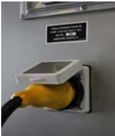
Exterior RV Style Electrical Cord Hook-Up
