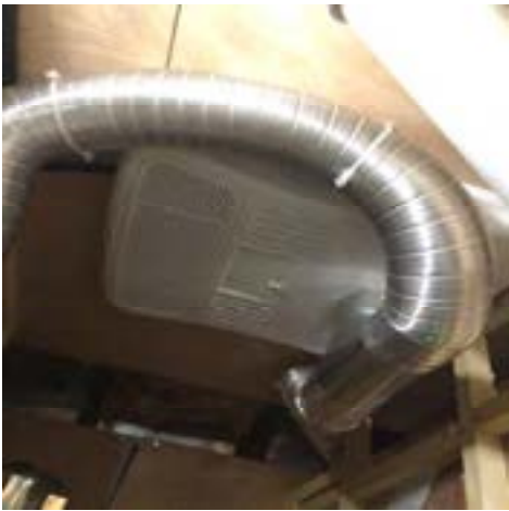
Roof A/C and Ducts
