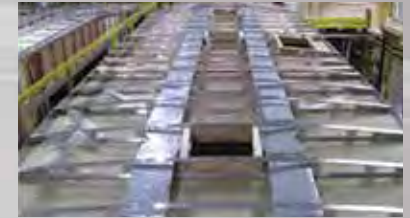
3" Aluminum floor studs, heat duct and 5/8" tongue and groove plywood floor.
