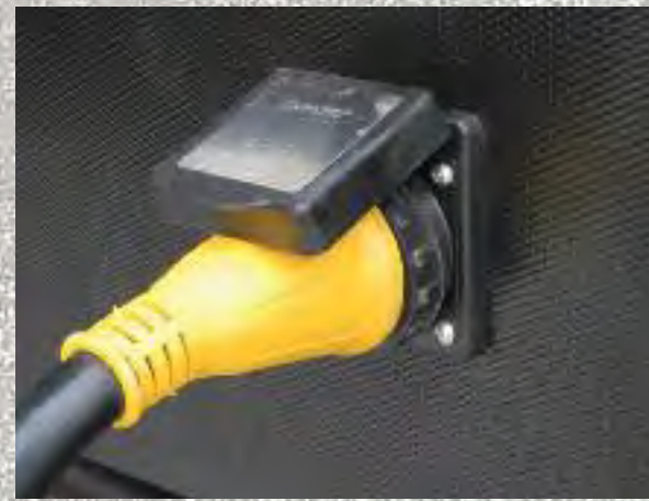
30 AMP Service with Transfer Switch
