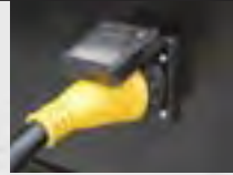
50 AMP Service with Transfer Switch
