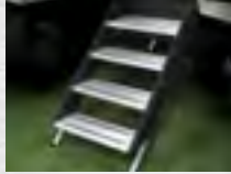
Upgraded Quad Main Entry Steps
