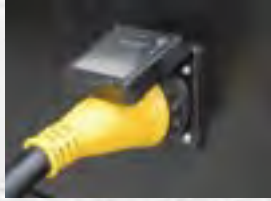
50 AMP service with transfer switch
