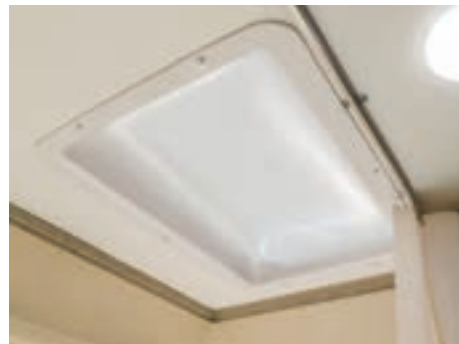
Skylight over Tub
