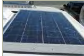
ROOF SOLAR PANEL PREP
