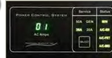
ENERGY MANAGEMENT SYSTEM - CAN RUN 2 A/C'S ON 30 AMP & 3 A/C'S ON 50 AMP
