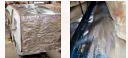
R-38 Radiant shield Thermo-foil wrap through ceilings, underbellies and under front cap.
