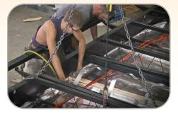
Competitors install a one piece underbelly design which is screwed into the frame.
