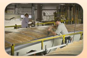
A full length 3/8" wood decking, for a full walkon roof, is screwed, not stapled, into place. Our final step is adding a twoply, Tuff ply<sup>™</sup>, rubber roof membrane with a built-in fire retardant and 12 year warranty.
