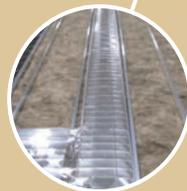
Water lines are insulated within the floor substrate, not below the floor.
