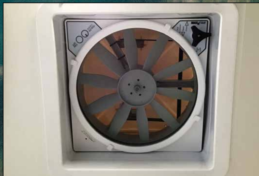
High Output Attic Fan in Bathroom
